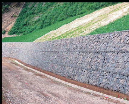
Mountainside soil-retaining construction / Retaining wall
