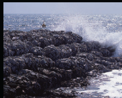
Harbor Embankment Mat Construction
