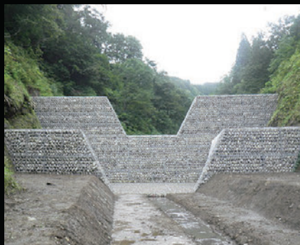
Erosion Control Construction
