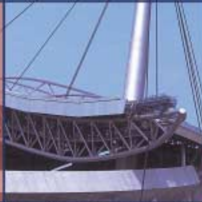
Hanging Roofs Structure
